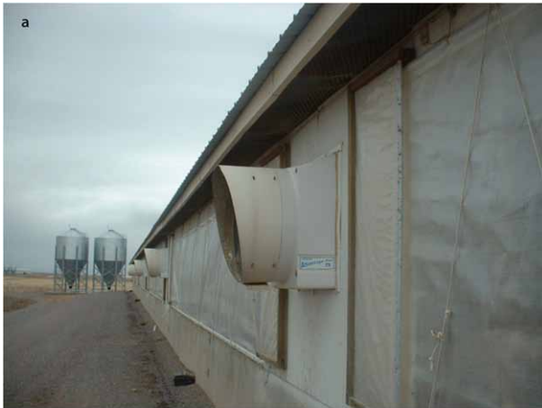
Figure 11.4. Modern-day mechanical ventilation system with sidewall fans for ventilation control.
