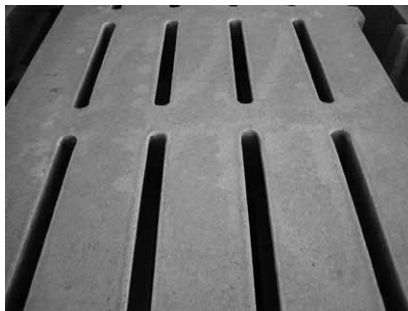
Figure 17.4. Slatted concrete floors, when well designed, constructed and maintained are a good pavement for obtaining clean and healthy livestock (photo: Anses, Ploufragan).
