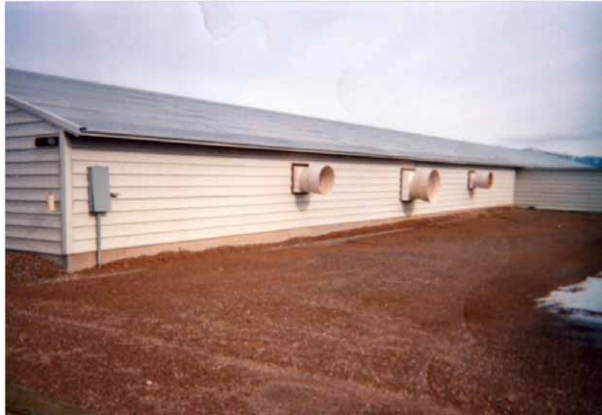
Figure 11.4. Modern-day mechanical ventilation system with sidewall fans for ventilation control.
