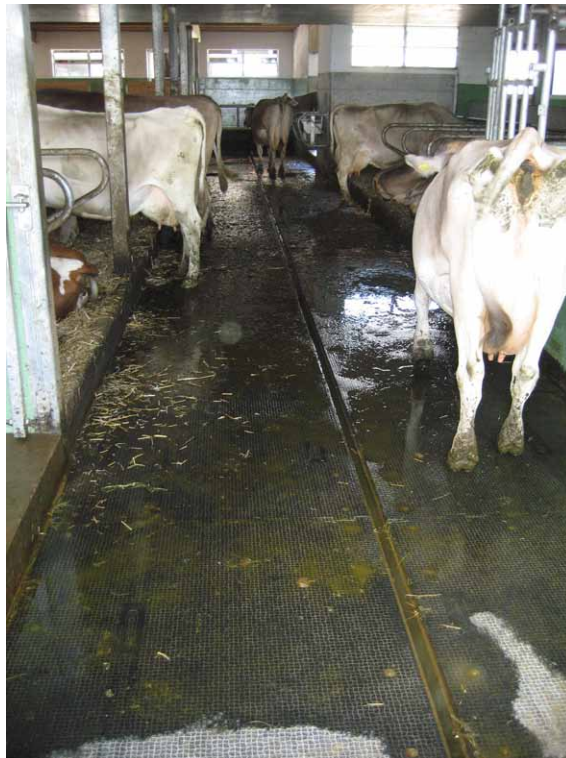
Figure 4.2. Rubber flooring in passage way for dairy cattle.
