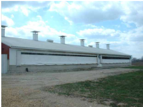
Figure 11.3. Naturally ventilated pig building with chimneys and sidewall curtains with split-zone control of one room.
